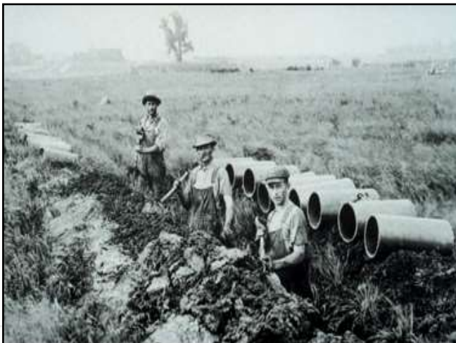
Hand digging tile, Boone Co. IA, ca 1914 Source: 'An Iowa album: a photographic history, 1860-1920' by M. J. Bennet, University of Iowa Press, Iowa City, Iowa
